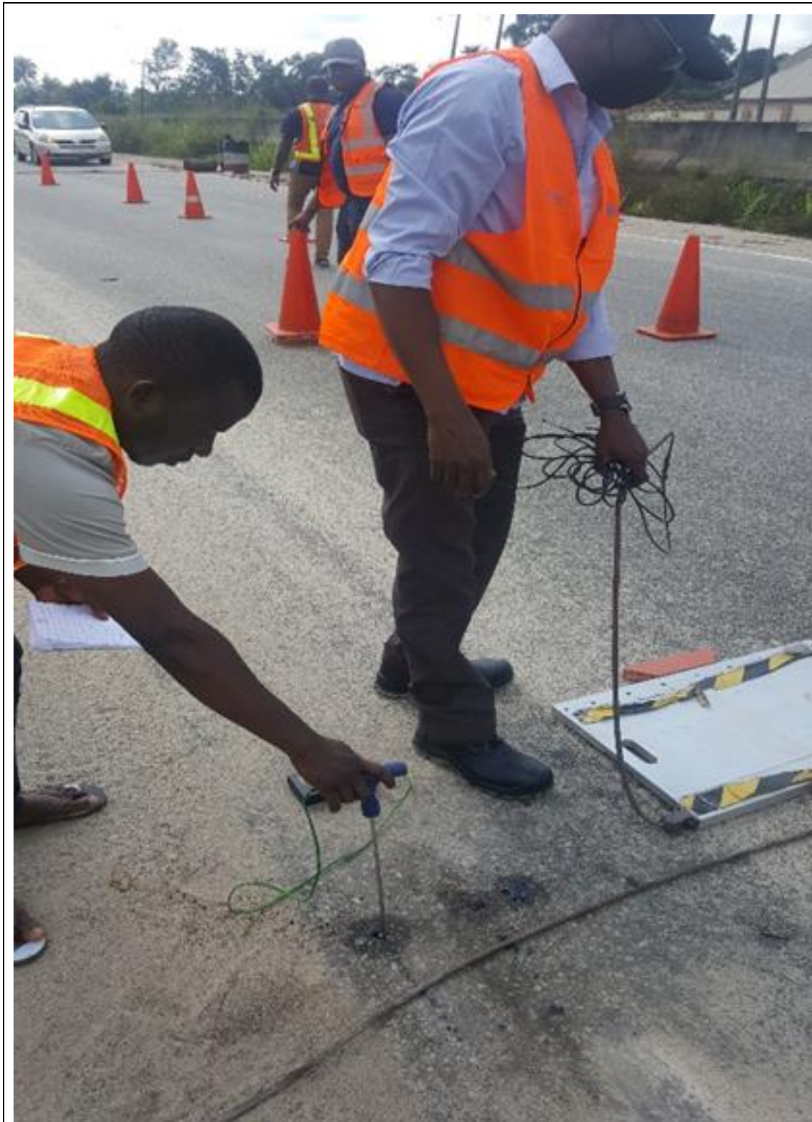
Figure 7 Pavement Temperature testing
