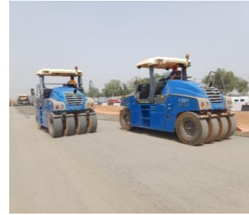
Compacting of BSM
