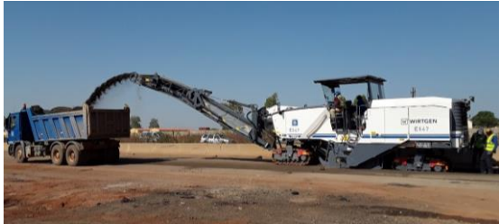
Milling of existing road structure (RAP and GBC material)
