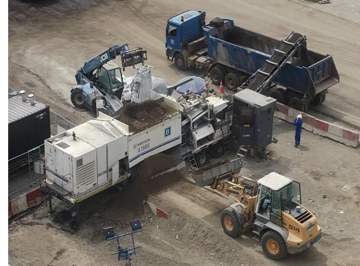
In-Plant Mixing (BSM production)
