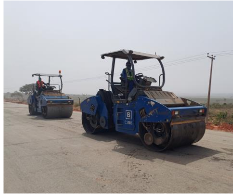
Compacting of BSM
