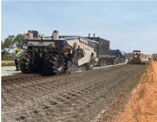
In-Situ: Milling and Stabilizing
