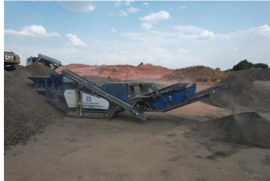
Preparation ( Crushing ) of milled material
