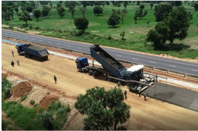
Paving of BSM
