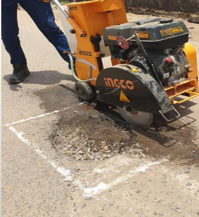
Cutting of pothole
