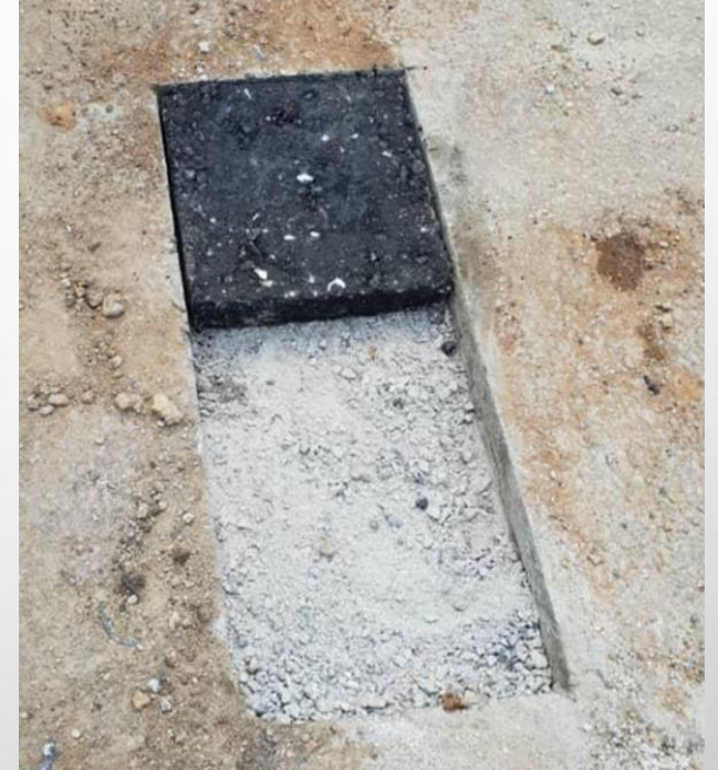
Test fitting of resized pothole
