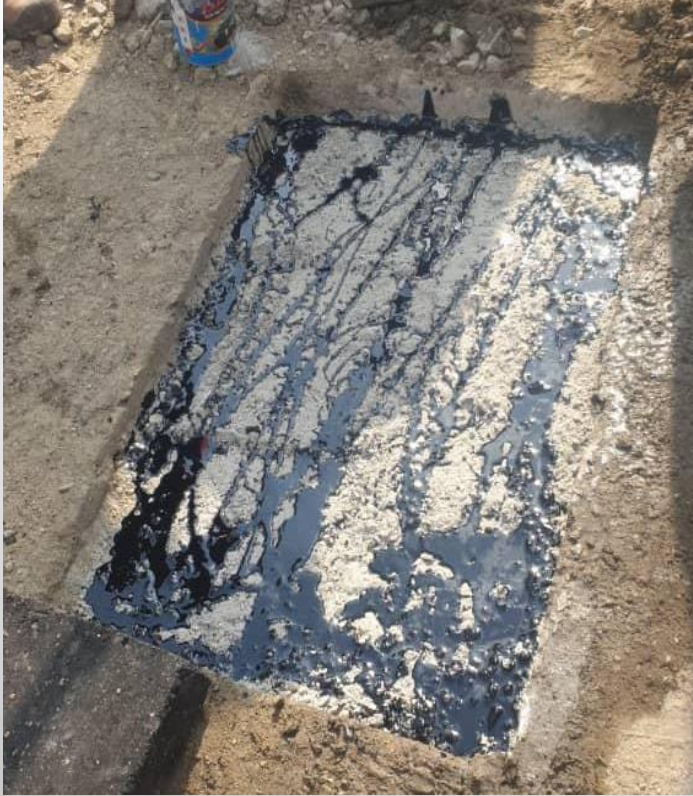
Priming of Pothole
