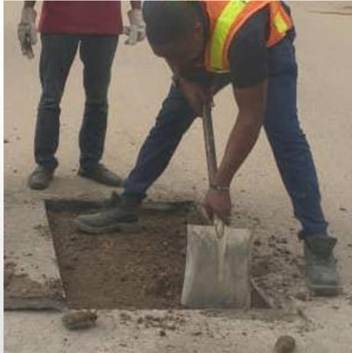
Scarification and cleaning of pothole
