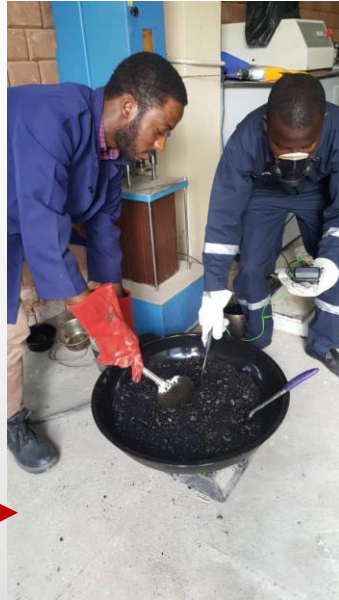
AGGREGATE AND BINDER MIXING
